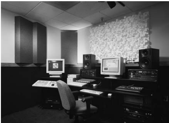
Figure 6.3 Top: Measured and predicted normal incidence absorption coefficient for a commercial membrane absorber (Modex™). Bottom: A typical installation in a small reproduction room, the absorber is in the corner of the room. (Photo courtesy of RPG Diffusor Systems, Inc.)
