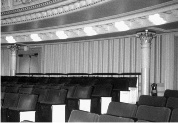
Figure 2.1 Schroeder diffusers (QRD®s) applied to the rear wall of Carnegie Hall to prevent echoes (after D'Antonio and Cox 2 ).
