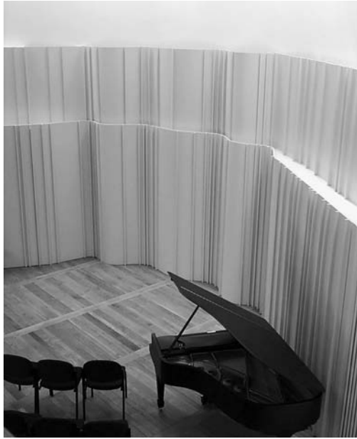
Figure 2.35 Optimized curved surface (OptiCurve™) in the Edwina Palmer Hall. (Photo courtesy of Arup Acoustics.)
