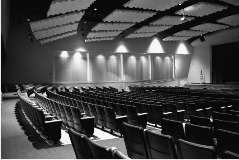
Figure 2.36 Optimized curved audience canopy (Waveform® Bicubic) in Patterson Mill Middle and High School, MD (CSD Architects, Baltimore, MD; photo courtesy of RPG Diffusor Systems Inc.)
