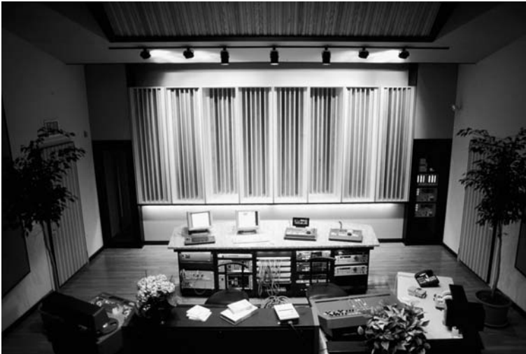
Figure 2.12 Gateway Mastering, Portland, ME, showing a fractal diffusing rear wall (Diffraactal®). (Photo courtesy of Gateway Mastering + DVD.)
