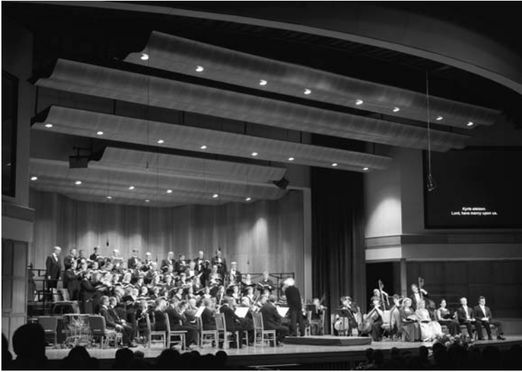
Figure 2.26 Rear towers and overhead stage canopy (Overture®) at First Baptist Church, Eugene, OR. (Photo courtesy of Steve Diamond, AGI, Inc.)
