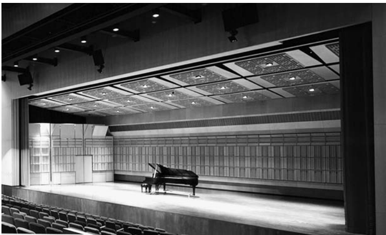
Figure 2.32 Diffusers around the stage of the Corning Glass Center, NY. (Photo © Paul Warchol Photography, www.warcholphotography.com )
