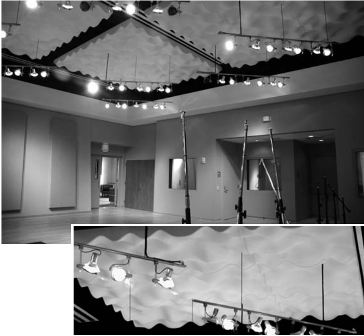
Figure 10.36 Modulated curved diffusers used in the ceiling of a radio production studio at KTSU, Texas Southern University, Houston, TX (Acoustician: HFP Acoustical Consultants). Insert shows close-up of ceiling.
