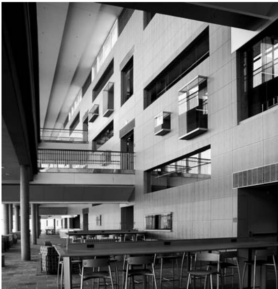
Figure 1.1 Perforated, absorptive wood panelling covering the entire feature wall opposite an exterior glass wall (out of shot) in Morgan State University in Baltimore, MD. (Acousticians: Shen, Milsom and Wilke, Ballston, VA. Photo courtesy of RPG Diffusor Systems, Inc.)
