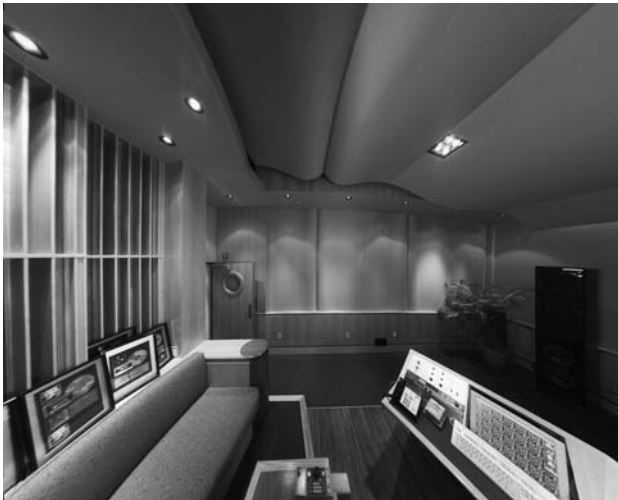
Figure 11.5 A curved hybrid diffuser applied to the ceiling and side walls of SonyM1, New York. (Photo by Paul Ellis of The M Network Ltd, Acoustician: Harris, Grant Associates.)
